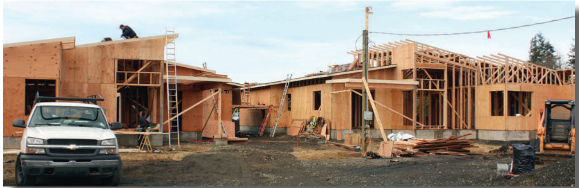
Work continues in January on phase 1 of the Tillamook subdivision.
