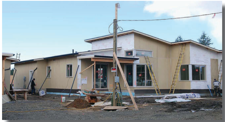
Construction progresses in March at the Tillamook subdivision.
