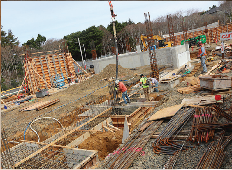
The parking structure in various stages of construction
