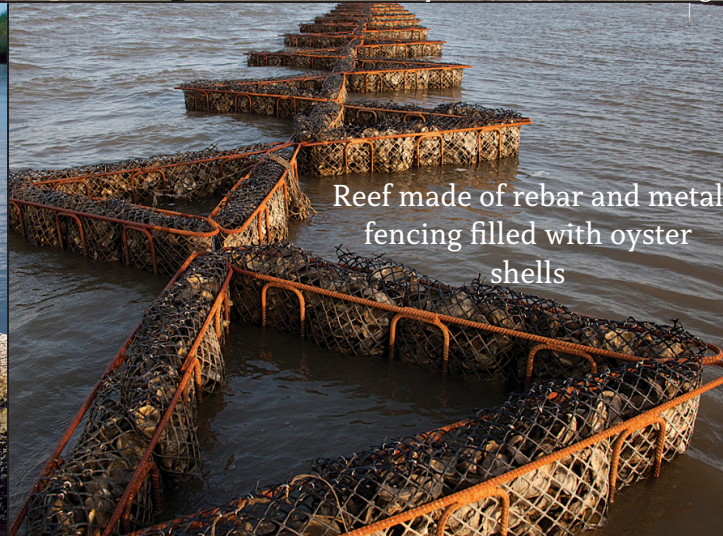
Reef made of oyster shells in mesh bags
